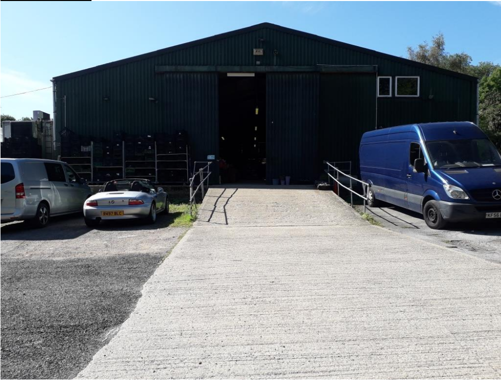
Front of existing warehouse building
